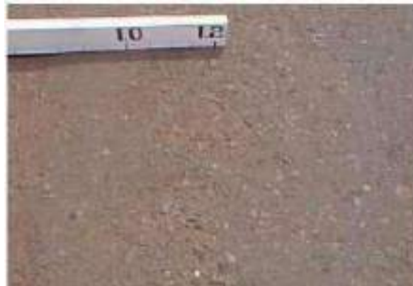
Gambar 2. 12 Pengausan Agregat ( Polished Aggregate )
