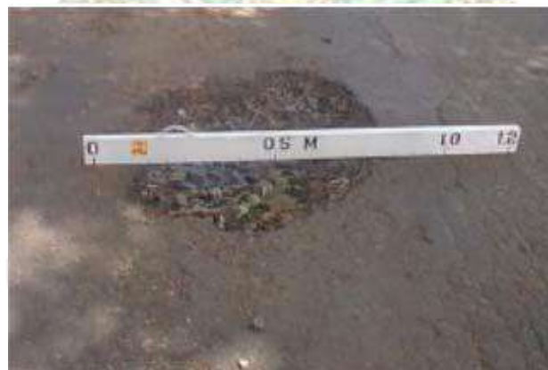
Gambar 2. 13 Lubang (Potholes)
