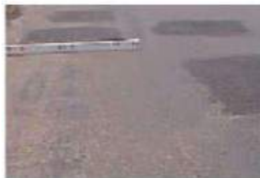
Gambar 2. 11 Tambalan dan Galian Utilitas ( Patching and Utility Cut Patching ) (Sumber: Bina Marga no.03/MN/B/1983)
