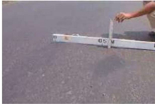
Gambar 2. 15 Alur ( Rutting ) (Sumber: Bina Marga no.03/MN/B/1983)
