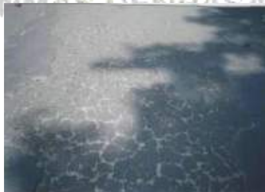
Gambar 2. 19 Pelepasan Butir ( Weathering/Raveling )
