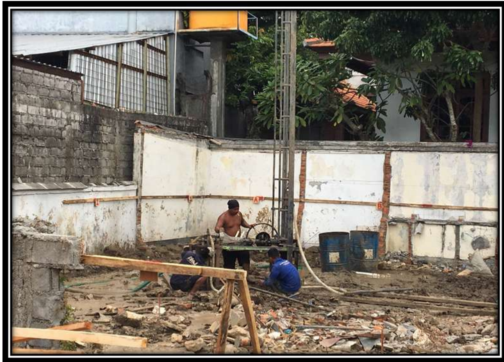
Gambar 2.6 Metode Basah ( Wash Boring Method )
