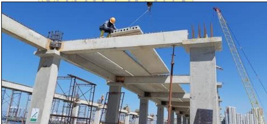
Gambar 2.11 Beton *Precast*
