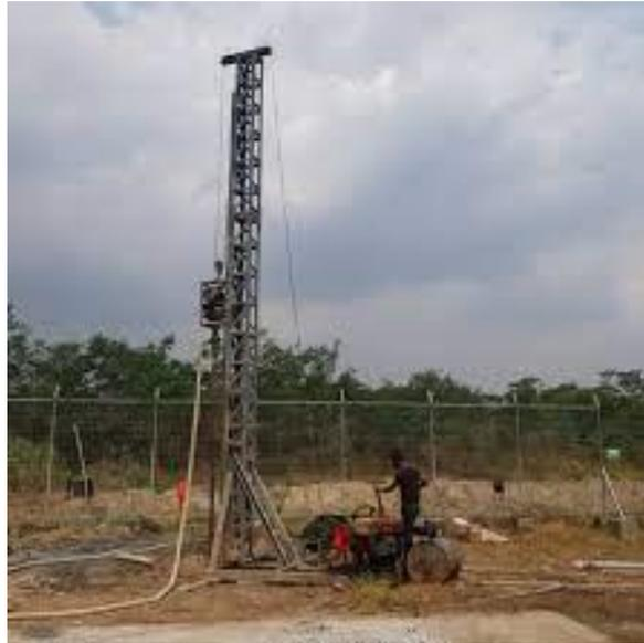
Gambar 2. 11 *Bore Pile Mini*
