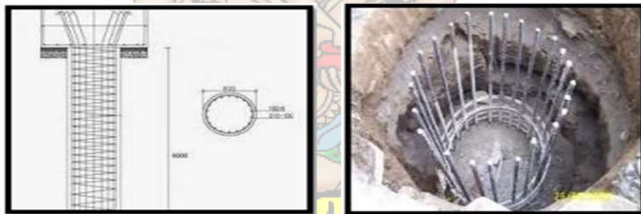
Gambar 2.18 Pondasi Bore Pile (Arsitur Studio, 2020)
