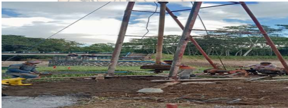
Gambar:2.20 Metode Basah ( wash boring method ) (Sumber : PT. Pramana Artha Raharja)
