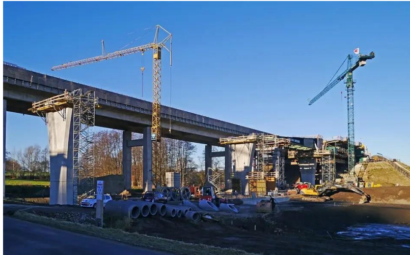
Gambar 2. 3 Proyek Konstruksi Teknik Sipil ( Heavy Engineering Construction ) (Dekoruma, 2018)
