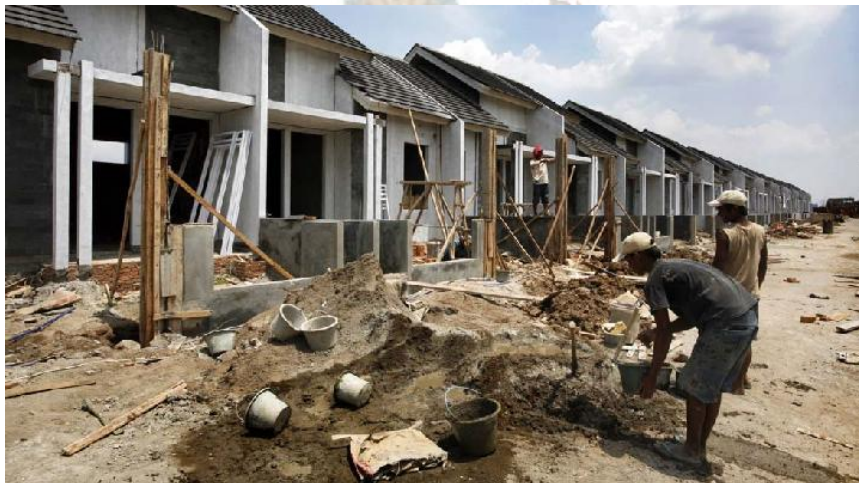
Gambar 2. 1 Proyek Konstruksi Perumahan ( Residential Constuction ) (Widyastuti, 2021)
