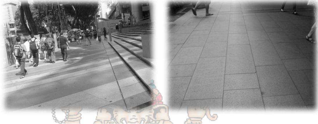
Gambar 2.30. Pola Lantai Miring Ukuran 40x80cm Material Andesit Abu abu,
